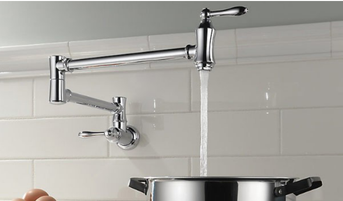
Pot Filler Pot fillers are cold water speciality faucets that come as either deck or wall mounted and are installed at the stove. The purpose of these faucets is for easy filling of pots that otherwise would be heavy or hard to carry from the kitchen sink. This is a great addition for those who love to cook!
